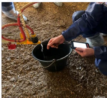
An endoscope, to inspect and verify the cleanliness of the water lines.
