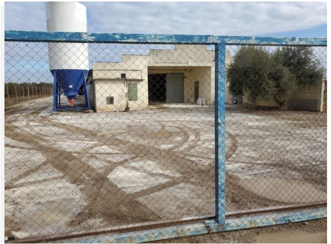
Figure 2. External area of the barn with calcium hydroxide.
