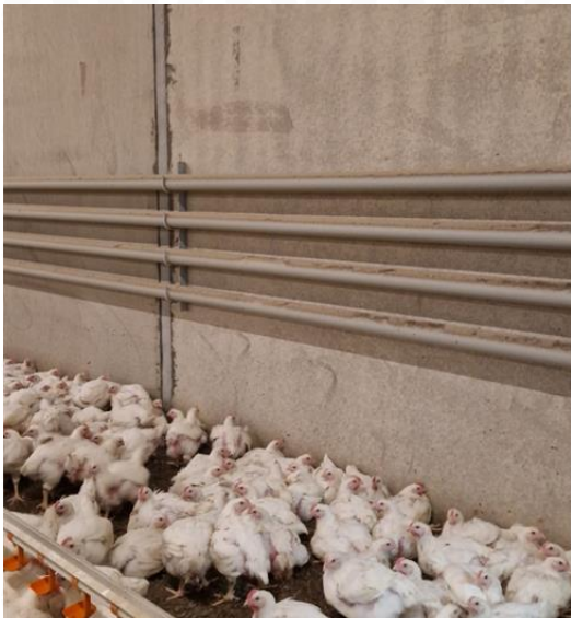
Radiators with circulating hot water ensure that the chickens always have the right temperature during rearing
